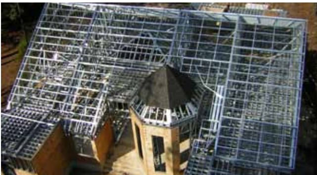
USA - Single Storey Residential Home
