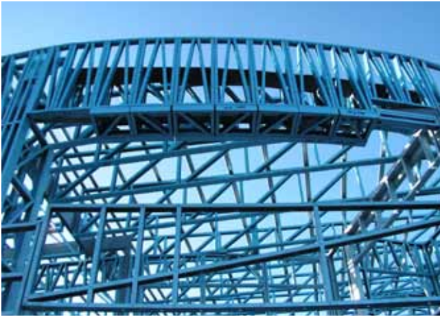
AUSTRALIA - Curved Truss System
