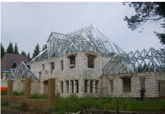
RUSSIA - Residential Roofing System
